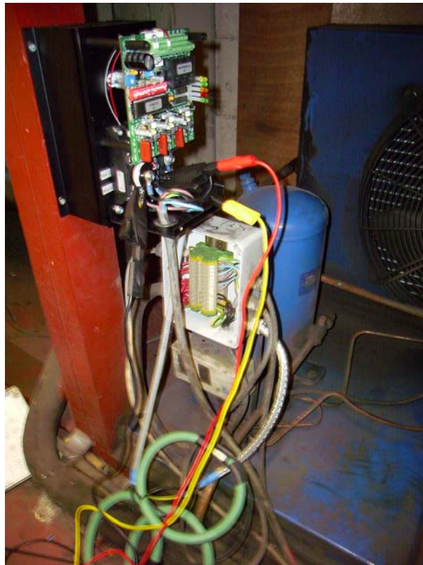
Figure 12: Three-phase EnviroStart MEC installation on walk-in freezer
