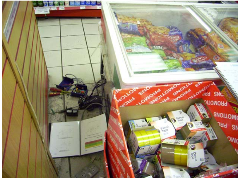
Figure 4: Chest freezer EnviroStart MEC installation
